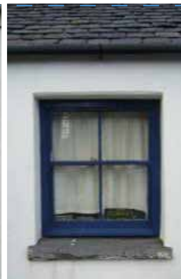
Window in keeping with the character of the area
